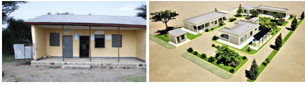
Figure 1: Basic health post (left); Design of a comprehensive health post that provides more essential services (right). Source: Ministry of Health, Ethiopia.
